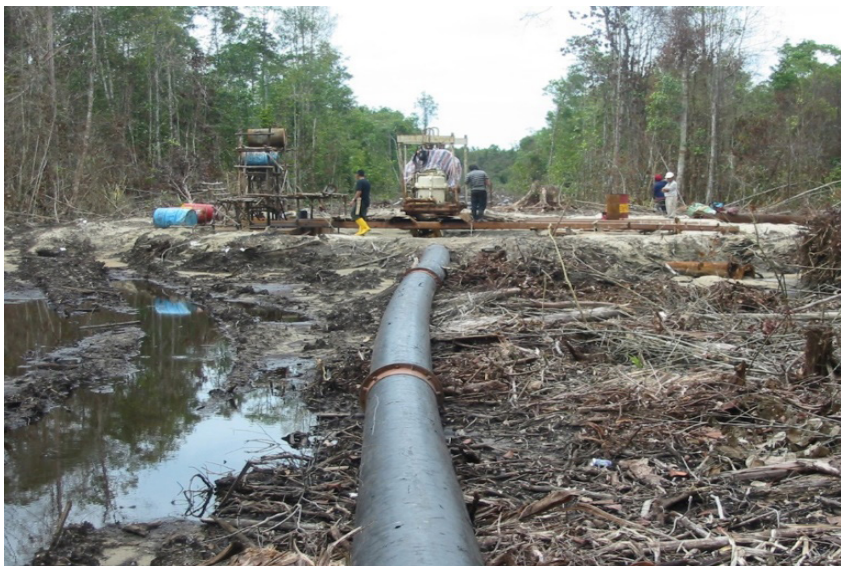
Figure 6 – 17. Hydraulic sand filling for Matang Highway, Kuching (Toh & Chee, 2000a)
