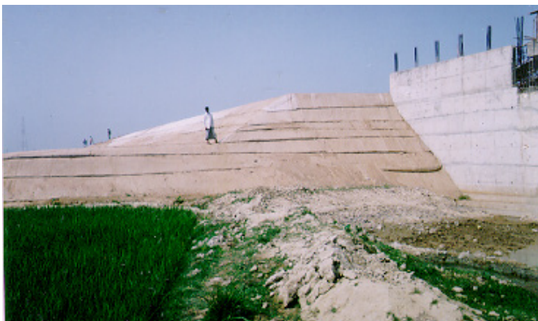
Figure 6 – 37. Manual placement of sand fill over reinforcement geotextile. Sylhet road, Bangladesh. (Toh & Chee, 2000b)
