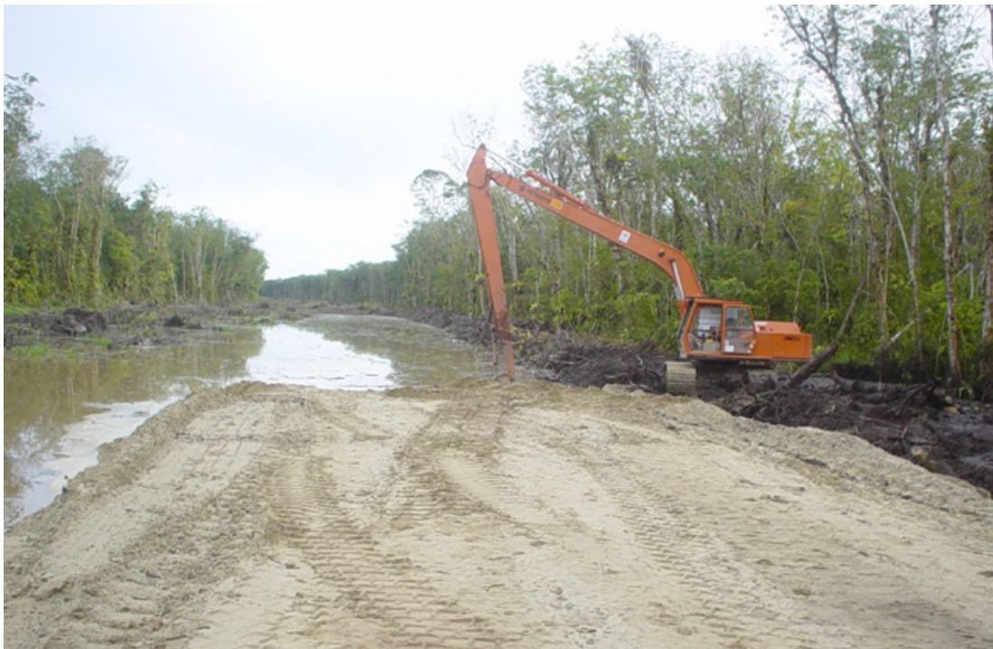
Figure 6 – 61. Excavation of peat without dewatering and backfilling with sand Jalan Nang Sang / Teku Link Road Sibul Sarawak. (JKR Sarawak and Hock Peng Furniture General Contractor) (2006).
