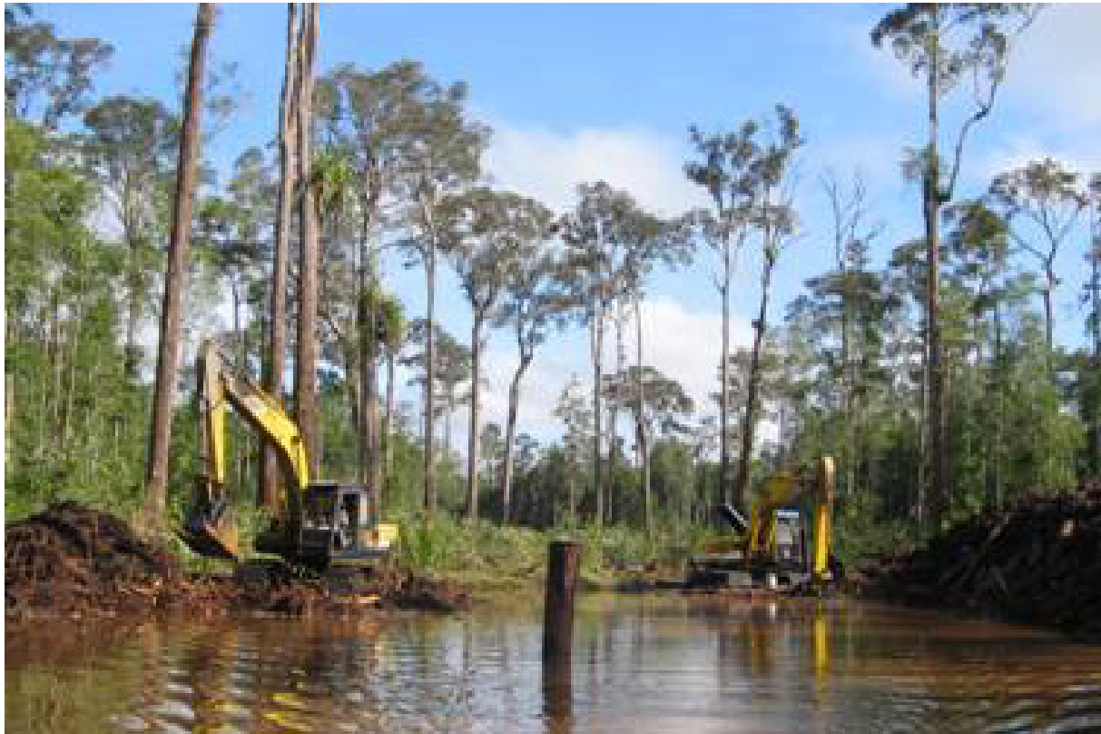
Figure 6 – 53. Peat excavation without dewatering for Sungei Bidut road, Sarawak. (Sarawak Construction & Jurutera Jasa, 2007)
