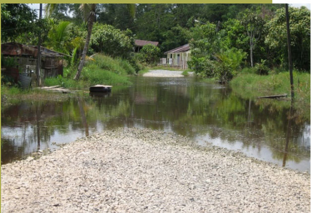
Figure 4 – 5. Excessive settlement and flooding of access road
