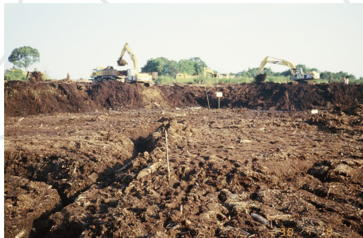
Figure 6 – 48. Excavation of dry peat at Machap, Johor. (Toh et al.,1990)
