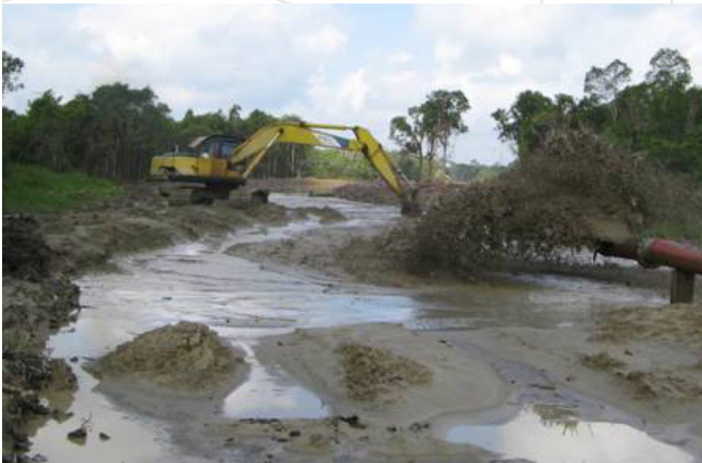
Figure 6 – 56. Pumping sand after excavation of peat for Sungei Bidut road, Sarawak. (Sarawak Construction & Jurutera Jasa, 2007)
