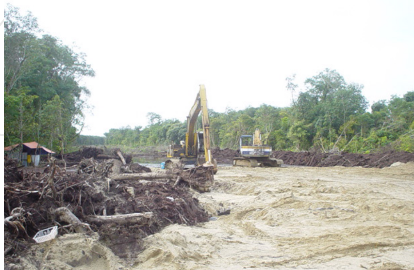
Figure 6 – 63. Sand fill contained by bunds formed using excavated peat. Jalan Nang Sang / Teku Link Road Sibul Sarawak. (JKR Sarawak and Hock Peng Furniture General Contractor, 2006)
