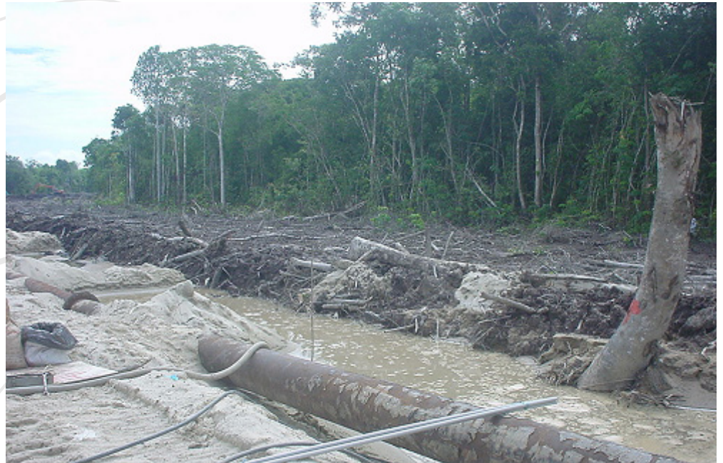
Figure 6 – 55. Pumping sand after excavation of peat for Sungei Bidut road, Sarawak.. Sarawak Construction & Jurutera Jasa, 2007)
