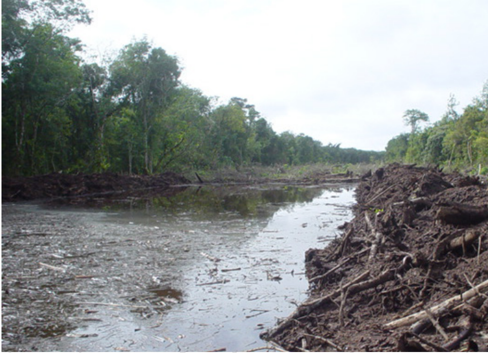
Figure 6 – 62. Excavation of peat without dewatering and use of peat as bunds for containing sand fill. Jalan Nang Sang / Teku Link Road Sibul Sarawak. (JKR Sarawak and Hock Peng Furniture General Contractor, 2006)
