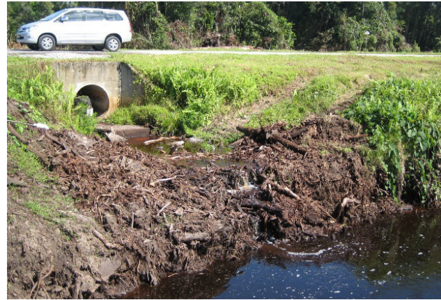
Figure 4 - 11. Lowered Ground water and ground next to pipe culvert
