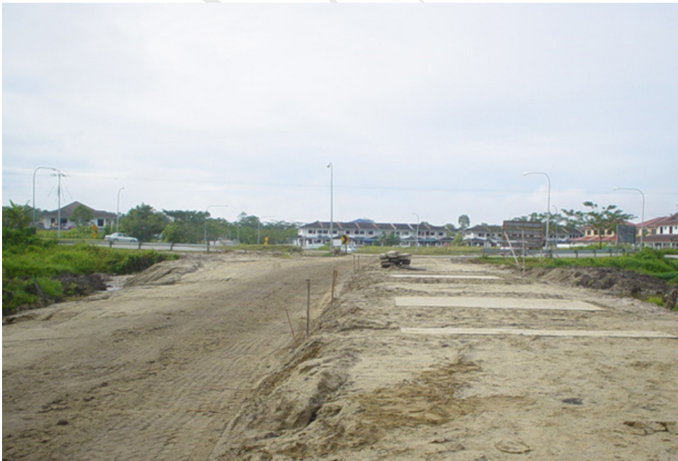
Figure 6 – 65. Completed sand embankment. Jalan Nang Sang / Teku Link Road Sibu Sarawak close to existing houses. (JKR Sarawak and Hock Peng Furniture General Contractor, 2006) General Contractor, 2006)
