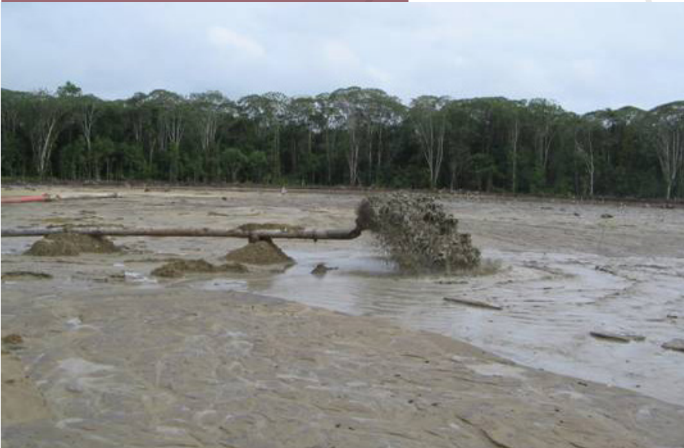
Figure 6 – 57. Pumping sand after excavation of peat for Sungei Bidut road, Sarawak. (Sarawak Construction & Jurutera Jasa, 2007)
