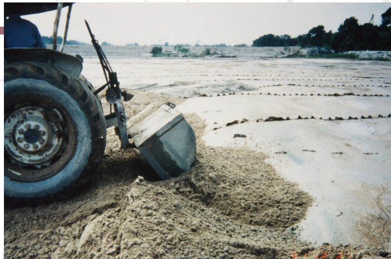
Figure 6 – 19. Filling over geotextile bamboo fascine mattress. (Toh et al 1994)
