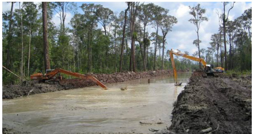
Figure 6 – 54. Peat excavation without dewatering for Sungei Bidut road, Sarawak. (Sarawak Construction & Jurutera Jasa, 2007)
