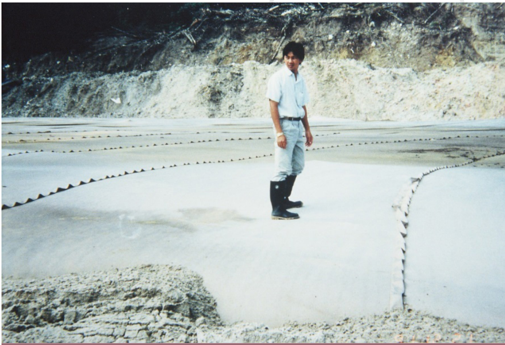
Figure 6 – 20. Mud wave ahead of filling contained by geotextile bamboo fascine mattress. (Toh et al 1994)
