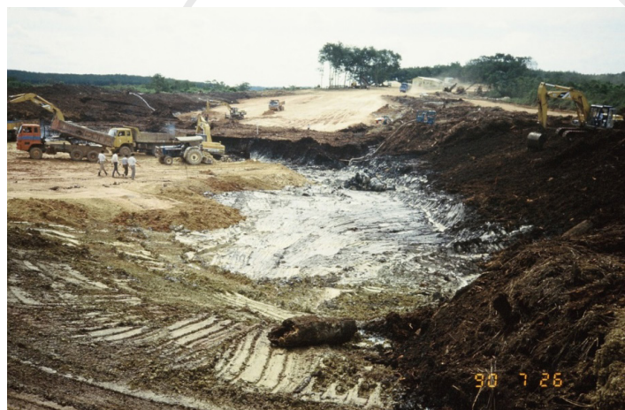
Figure 6 – 49. Excavation in dry and backfilling at Machap, Johor. (Toh et al.,1990)
