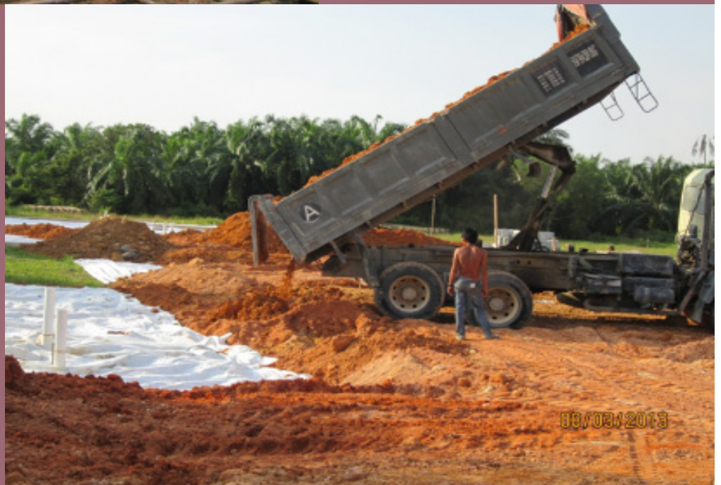
Figure 6 - 22. Placing fill over geotextile bamboo fascine mattress (photo courtesy of K S Low)
