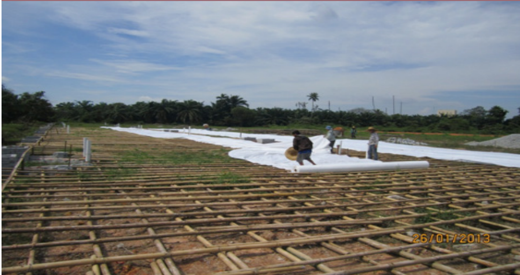
Figure 6 - 21. Placing geotextile over a bamboo frame on peat (photo courtesy of K S Low)
