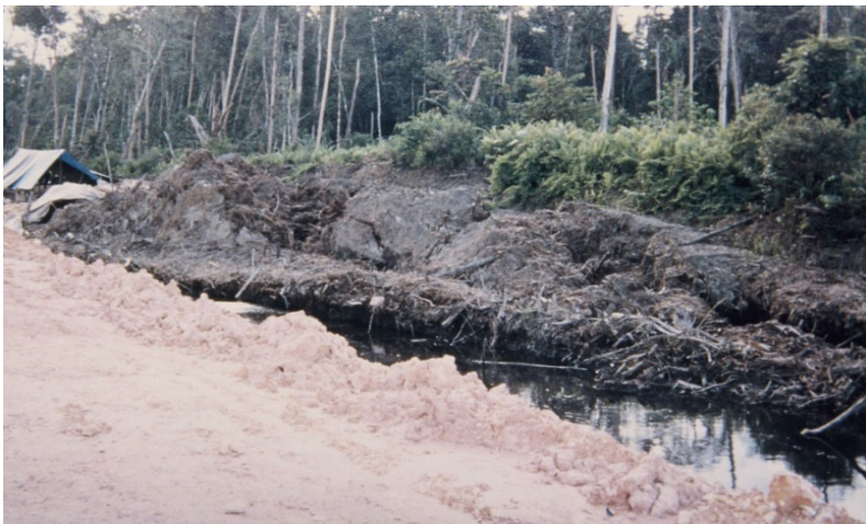
Figure 6 – 10. Heave during construction of the Air Baloi road, Johor. (Toh & Chee (2008))
