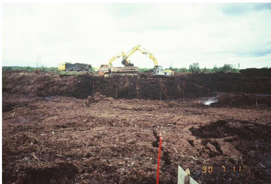
Figure 6 – 46. Excavation of peat and lowering of ground water at Machap, Johor. (Toh et al., 1990)
