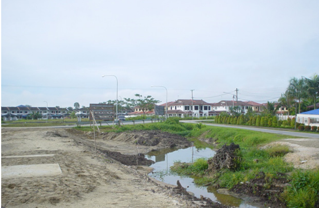
Figure 6 – 60. Jalan Nang Sang / Teku Link Road Sibul Sarawak close to existing houses. (JKR Sarawak and Hock Peng Furniture General Contractor) (2006)
