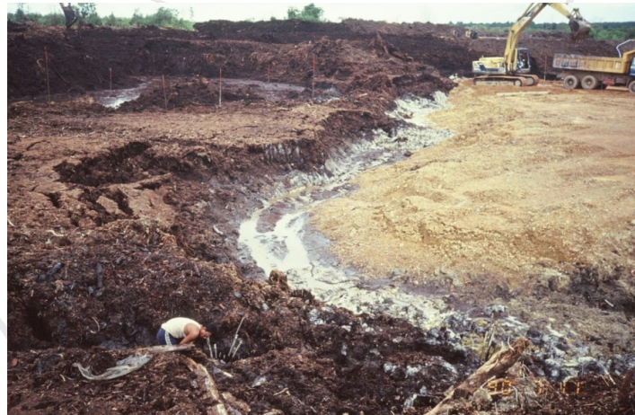
Figure 6 – 47. Excavation of peat with dewatering and backfill with residual soil in dry at Machap, Johor with compaction from (Toh et al.,1990)
