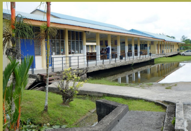
Figure 4 - 2. Ground settlement around a building founded on piles
