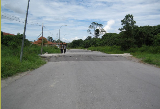
Figure 4 – 3. Settlement of road adjacent to culvert founded on piles
