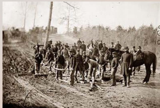
Figure 6 - 4. Corduroy road construction. American Civil War (from Google Images. 5 th October 2015)
