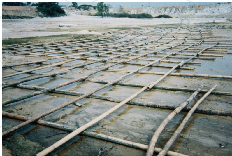
Figure 6 – 18. Bamboo frame for geotextile bamboo fascine mattress. (Toh & Chee, 2000b)
