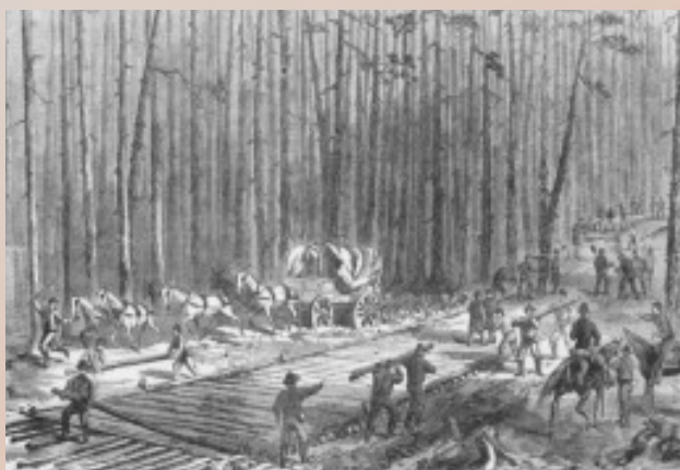
Figure 6 - 5. Corduroy road construction. American Civil war (from Google Images. 5 th October 2015)
