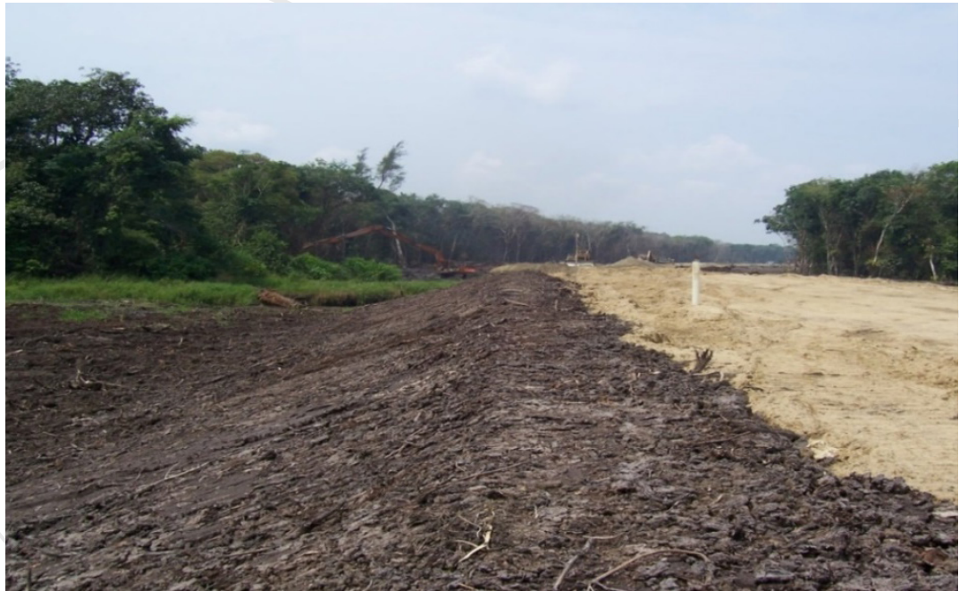
Figure 6 – 64. Sand fill embankment contained by peat bunds formed from excavation. Jalan Nang Sang / Teku Link Road Sibu Sarawak. (JKR Sarawak and Hock Peng Furniture General Contractor, 2006)
