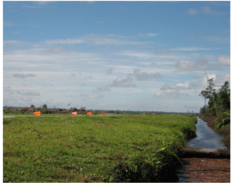
Figure 4 - 8. Lowering of ground water next to an existing road
