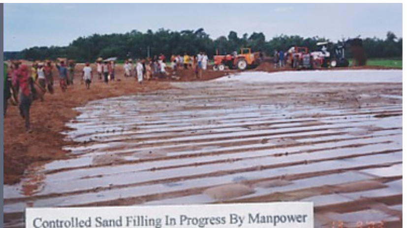
Figure 6 – 36. Reinforcement geotextile places over bamboo mattress for Sylhet road, Bangladesh. (Toh & Chee, 2000b)
