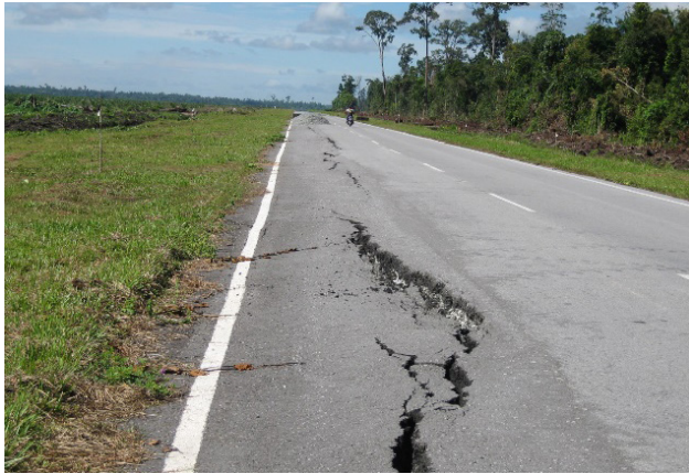
Figure 4 - 10. Damage to the road pavement due to agriculture with ground water lowering
