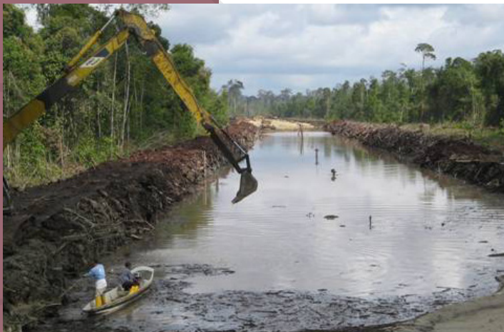
Figure 6 – 58. Excavated peat to form bunds to contain sand fill in embankment for Sungei Bidut road, Sarawak (Sarawak Construction & Jurutera Jasa, 2007)
