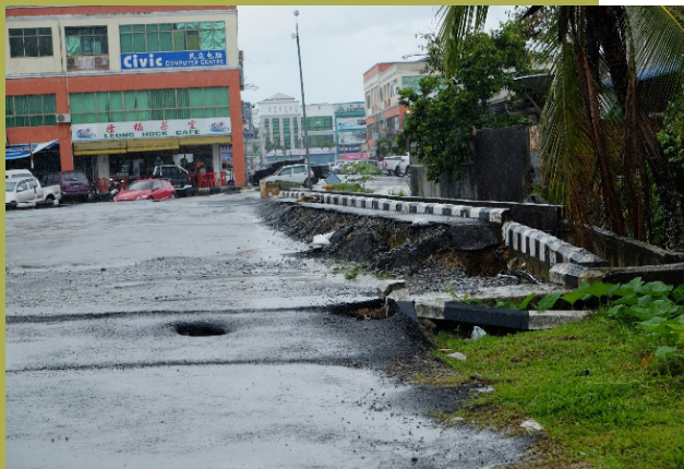
Figure 4 - 4. Settlement next to concrete drains supported on piles
