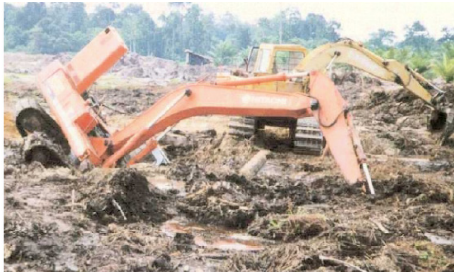
Figure 6 – 11. Excavator sinking into saturated peat (Low, 2015)
