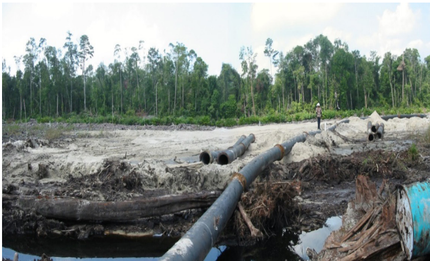
Figure 6 – 16. Hydraulic sand filling over peat swamp for Matang Expressway, Kuching. (Toh & Chee, 2000a)
