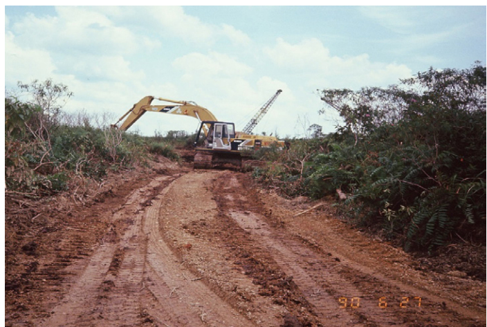
Figure 6 – 15. Drained peat surface after dewatering from nearby excavation (Toh & Chee, 2000a)
