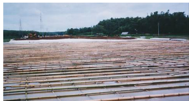
Figure 6 – 35. Geotextile bamboo fascine mattress for Sylhet road, Bangladesh. (Toh & Chee, 2000b)
